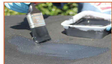
It is a dense liquid with a runny consistency and although can be polished off bodywork, you need to take a bit of care when applying it if you want to avoid unsightly black specks everywhere. The product smells like the stuff your mum used on your school canvas plimsolls back in the day. Once again, you need to brush it on, starting from the centre. The label says apply two coats, although we went for the belt and braces approach and applied three, leaving about 30-minutes between each one. The product becomes a little harder to work into the material with each progressive coat. Make sure you work it well in.
