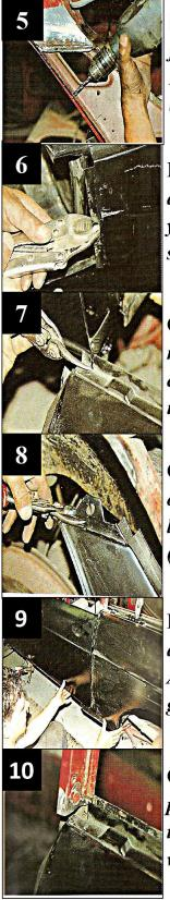
**SPOT WELDS:-** Drill out the holes in the rear inner wing/support frame so the new panel could be plug-welded from underneath. Don't worry about sticking to original weld positions, these varied during production.
