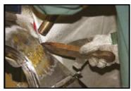
**9.** These blobs are then heated on the panel and pushed into the crevice with a wooden paddle dipped in tallow to keep it lubricated. The outer surface can be built up with more applications of the lead stick if needed, or the lead deposits moved around by heating them and pushing with the paddle.
